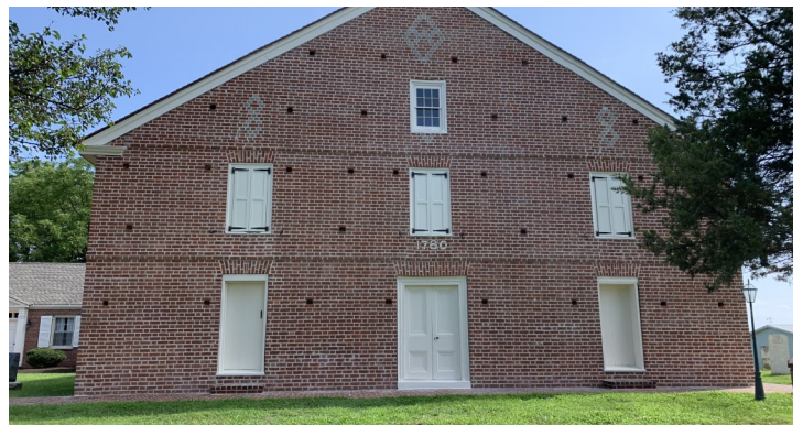
Photo taken 2020 following completion of repointing
